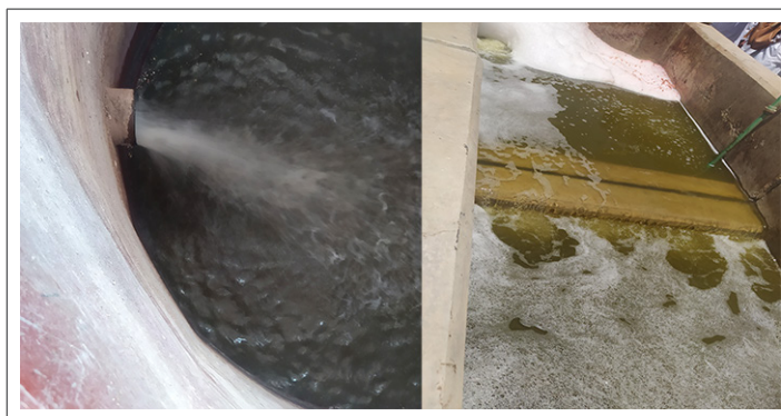
Figure 1. Wastewater inlet and outlet
